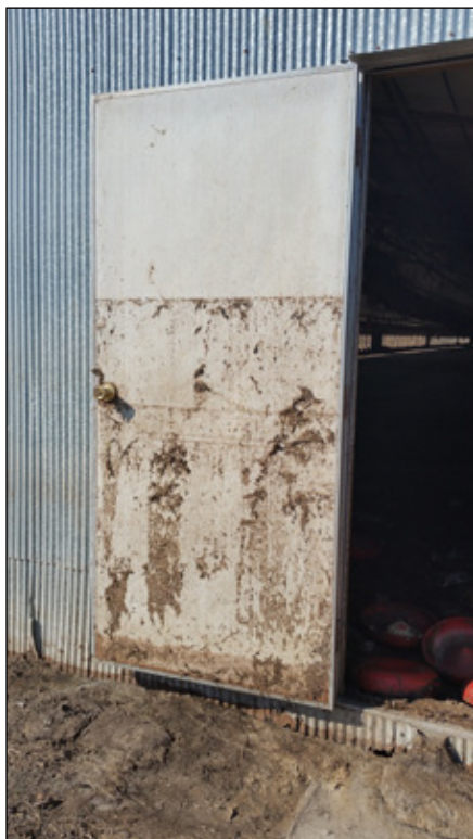
Fig. 5. Level of floodwater seen on a poultry house door (Source: Gary Flory, 2018).
